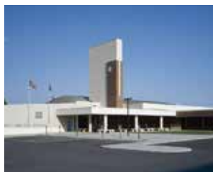
Crawford County Courthouse Adaptive Re-Use Pittsburg, KS
