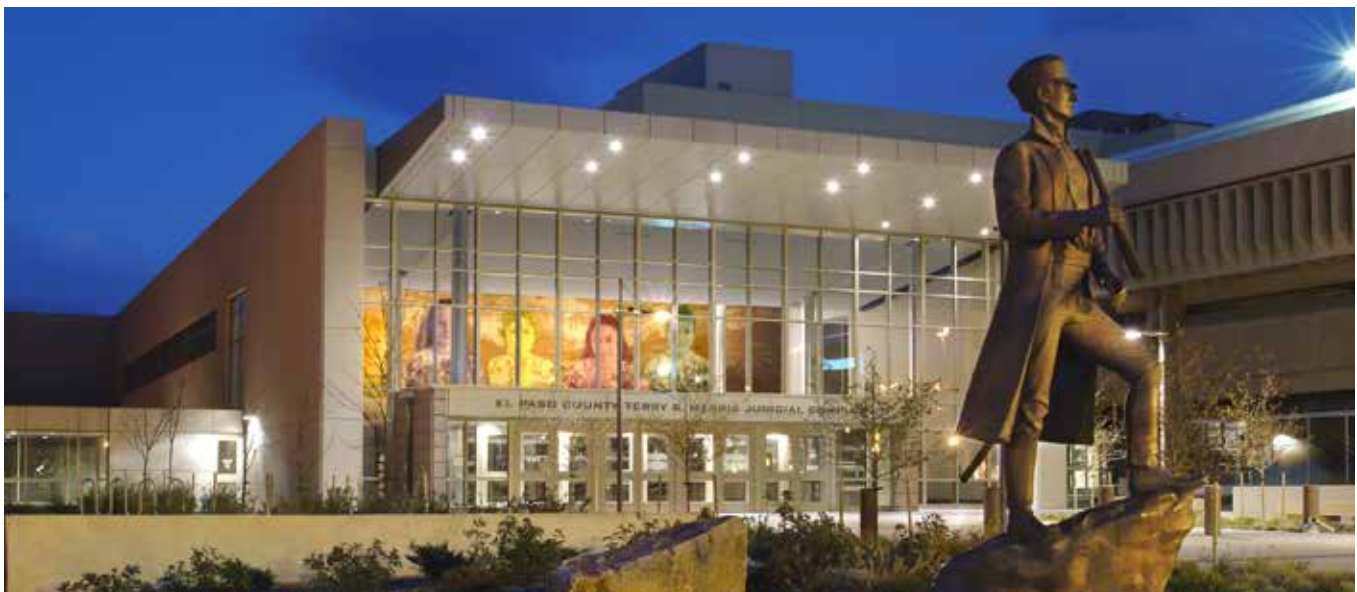
El Paso County Courthouse Expansion - New Entry Pavilion
