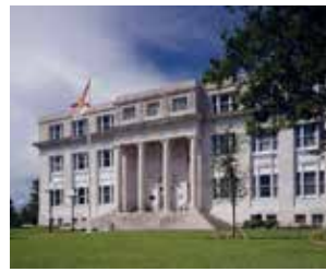
Highlands County Courthouse Expansion Sebring, FL
