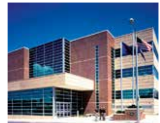
La Crosse County Justice Center and Courthouse La Crosse, WI
