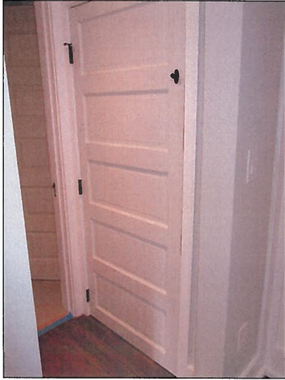
Figure 13: Typical restored interior door
