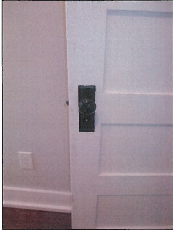
Figure 14: Typical restored interior door hardware
