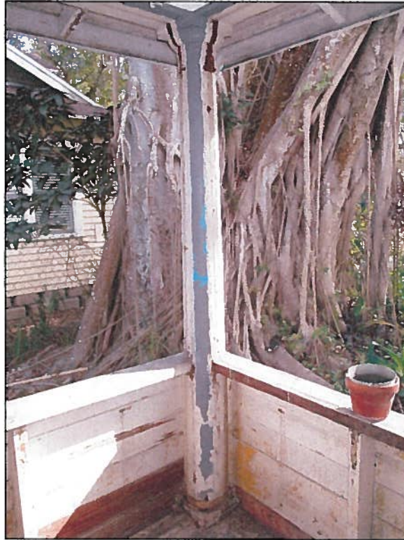
Figure 9: Column and rafter ends revealed by removal of porch enclosure
