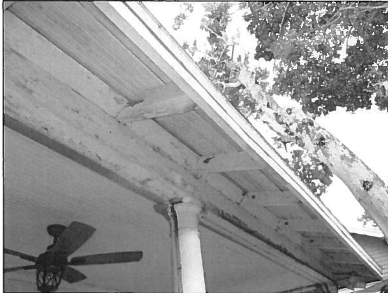
Figure 6: Restored and sistered rafter ends at opened cornice, porch column
