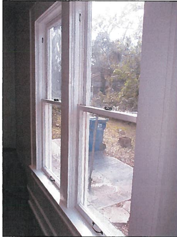
Figure 3: Typical restored windows from living room interior
