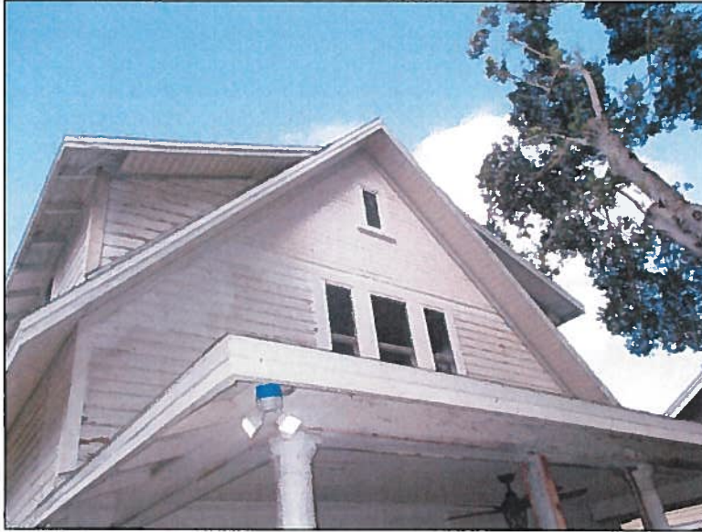
Figure 11: Original and replacement wood siding following removal of vinyl
