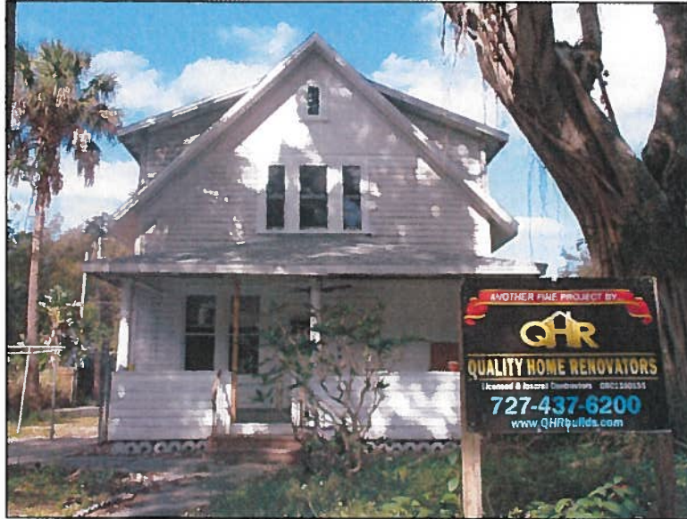
Figure 1: Façade (south elevation) of property at 823 10 th Ave. S., post-construction
