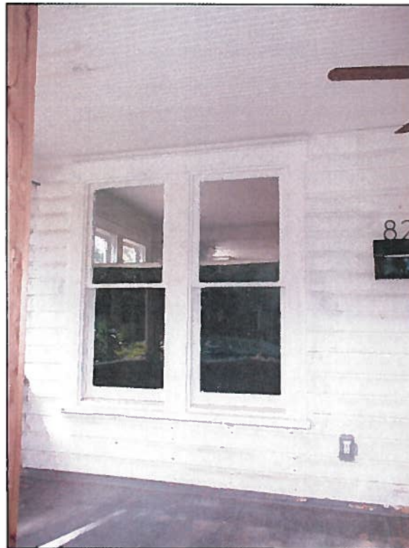
Figure 2: Typical restored windows at newly-reopened front porch
