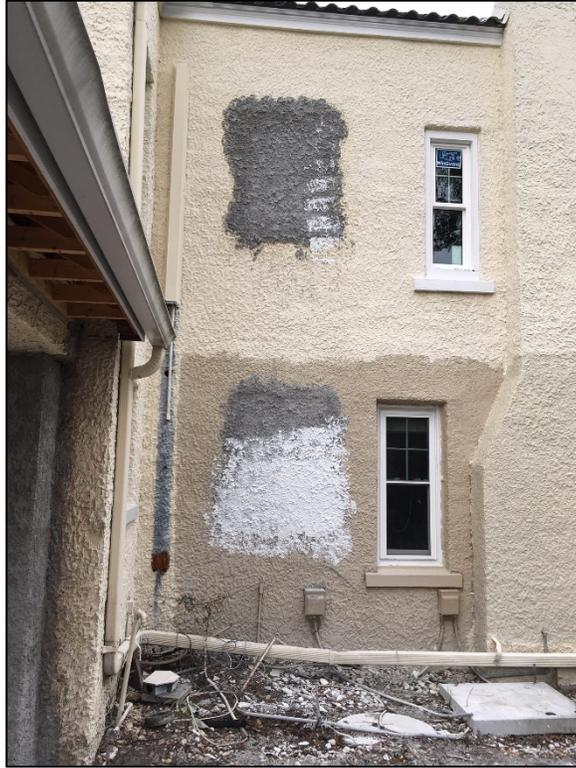
**Figure 11: Removed glass block windows and new window replacements**
