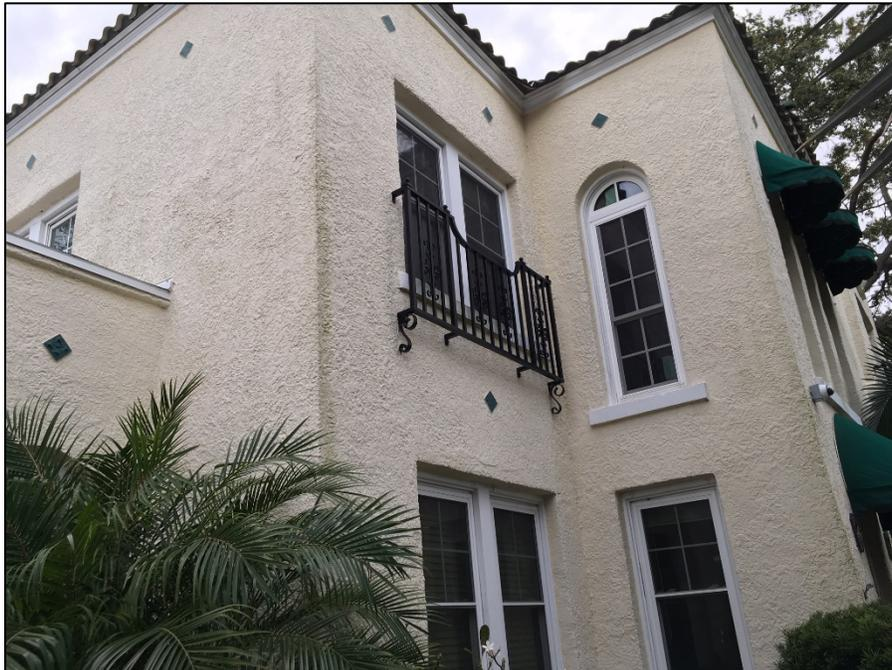
**Figure 14: Elevation showing replacement windows**
