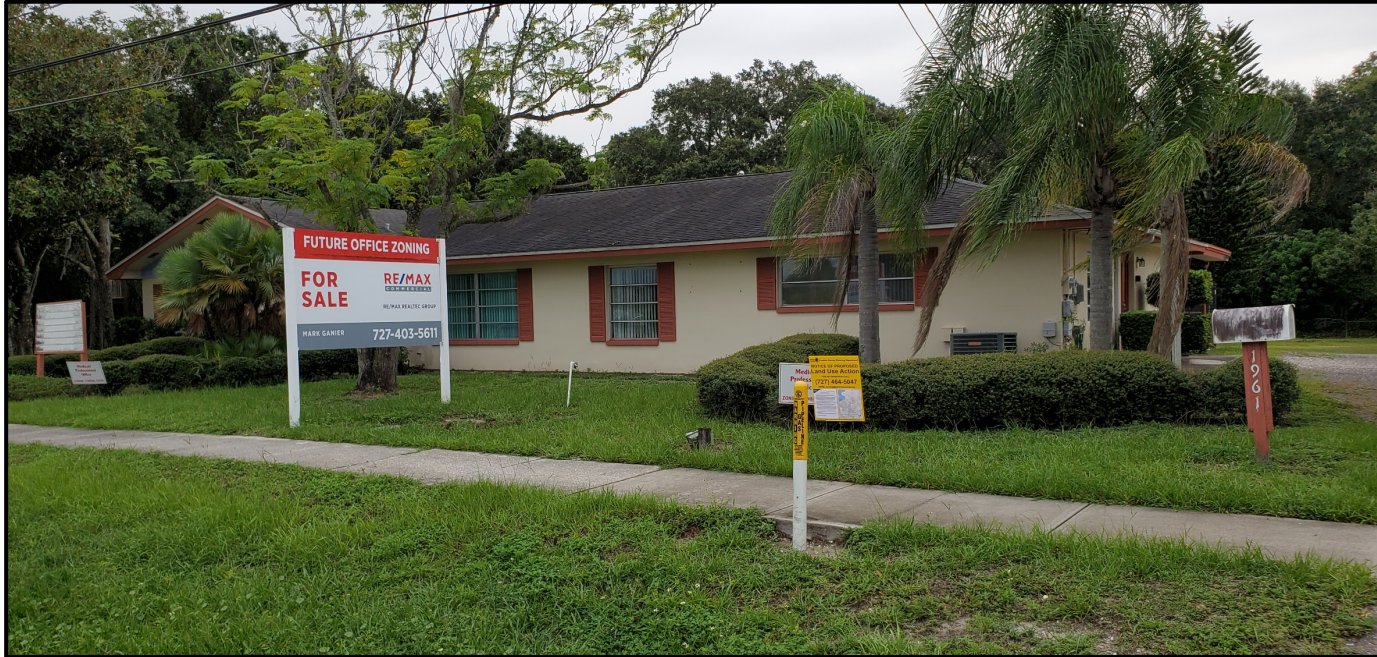
Looking east at existing building from East Lake Road
