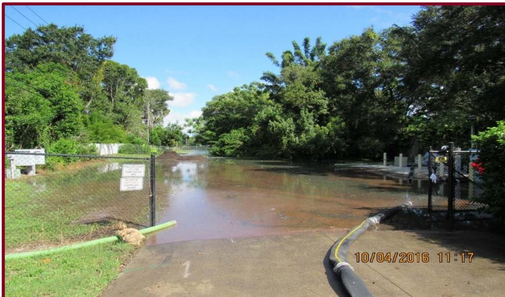
were already on-site responding to the issue. We observed that the sewer line break caused sewage to spill out in the retention pond, almost to the sidewalk by the Utilities pumping station. The smell emerging from the break was very toxic; in addition, there was heavily soiled greenery by the street.
