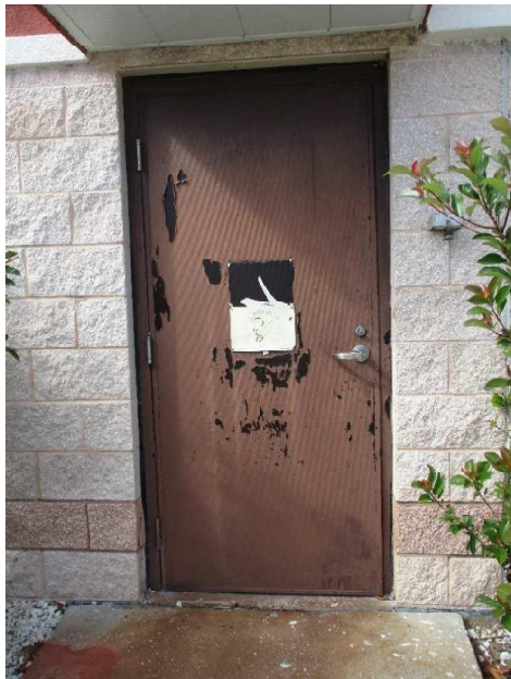
Photo No. 10 – Existing exterior metal doors
