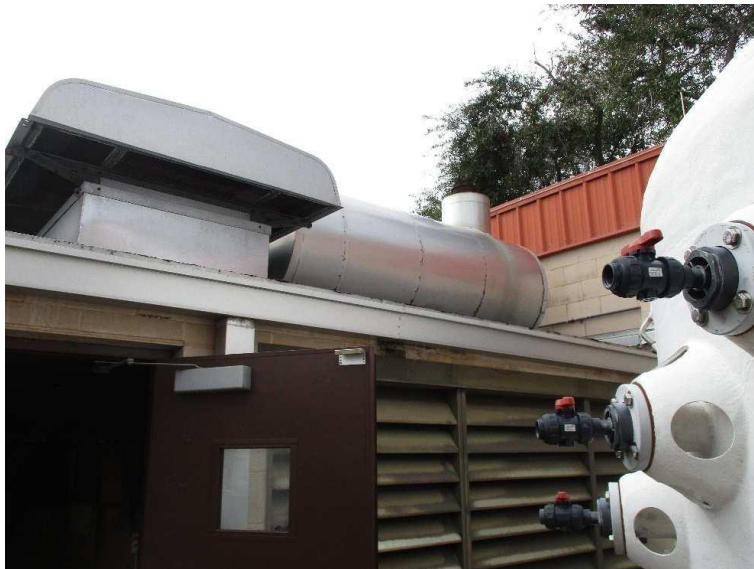
Photo No. 8 - North Louvers
