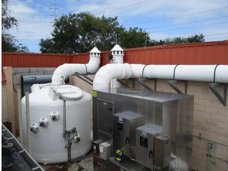
Photo No. 9 - Existing CMU Screening the Odor Control System
