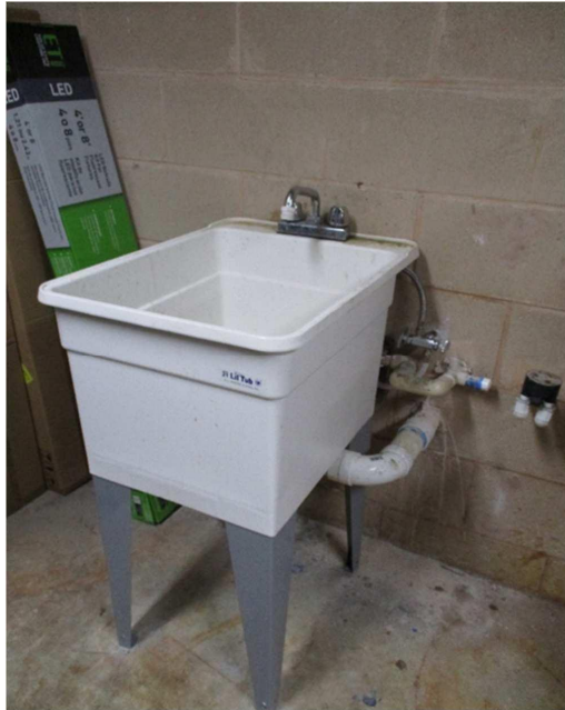
Photo No. 15 – Existing plumbing in northwest corner of chemical room
