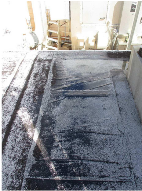
Photo No. 11 – Existing roof membrane over chemical room
