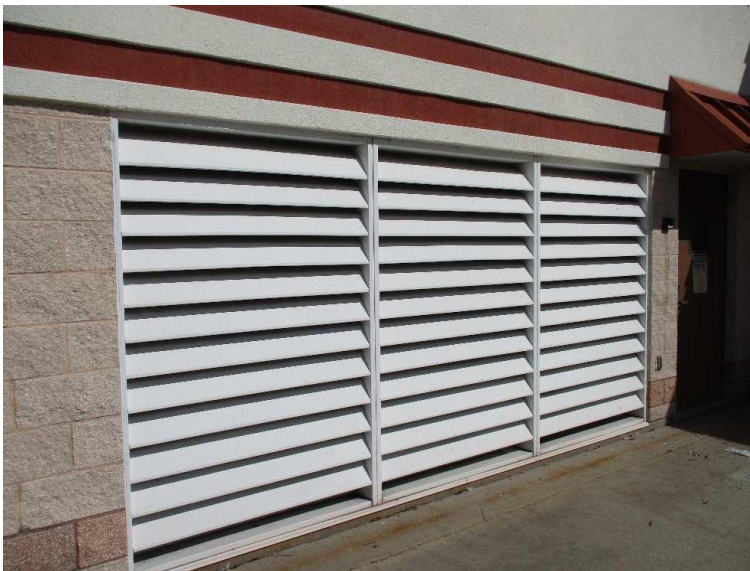
Photo No. 6 - Louver and Man- door, Southwest wall
