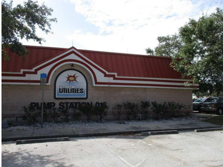
Photo No. 3 - North CMU Screen Wall
