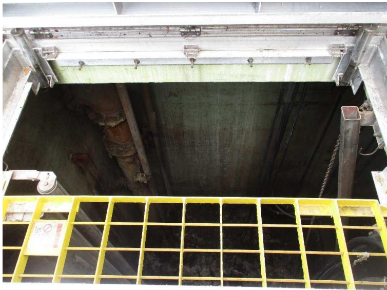
Photo No. 4 - Existing Wetwell Coating Example
