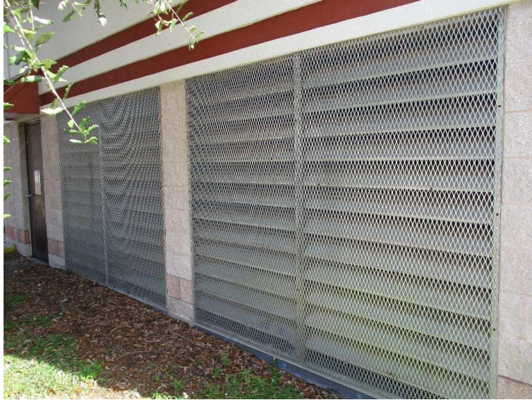
Photo No. 7 - Louvers, West wall
