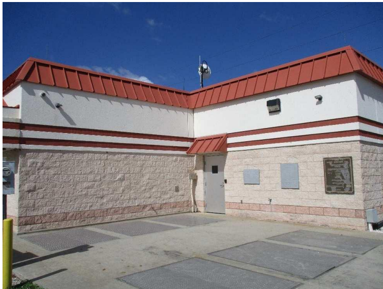
Photo No. 2 – East side Wetwell and Valve Vault Top Slab and Hatches and Man-Door to Odor Control Room
