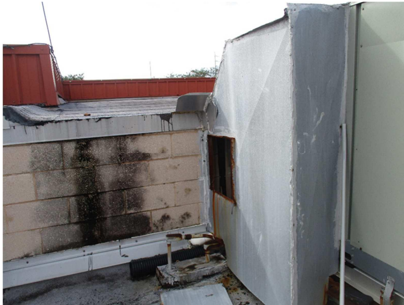
Photo No. 13 – Existing exposed CMU wall at roof change in level
