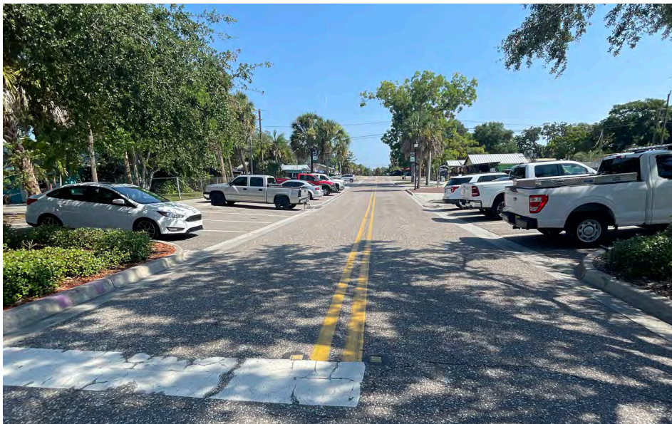
Existing Conditions: 11th Street and Florida Avenue looking north
