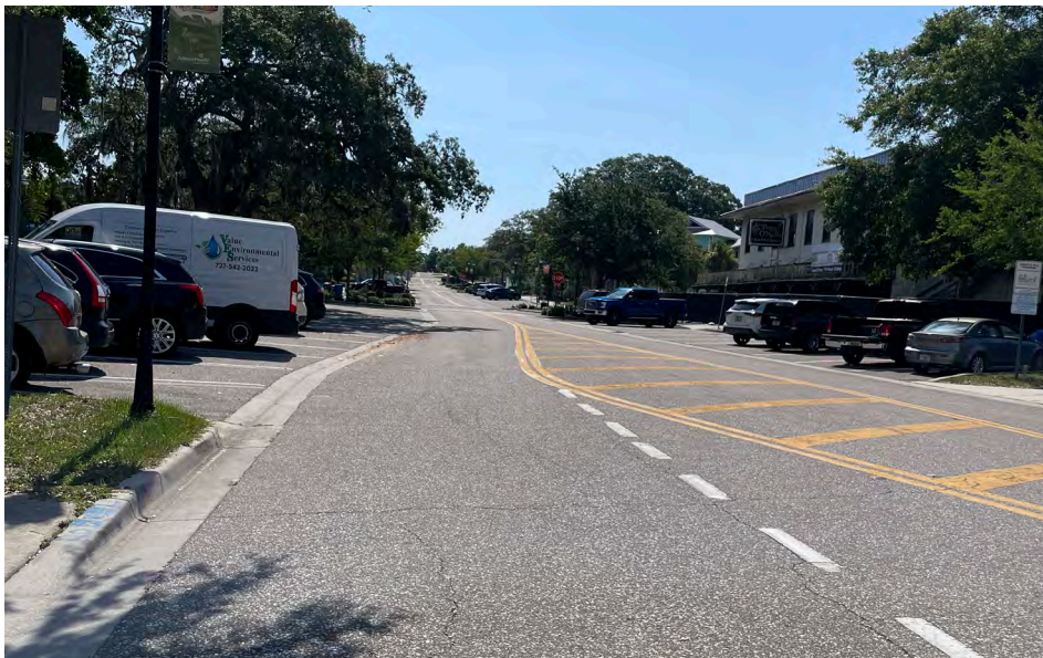
Existing Conditions: Florida Avenue looking east
