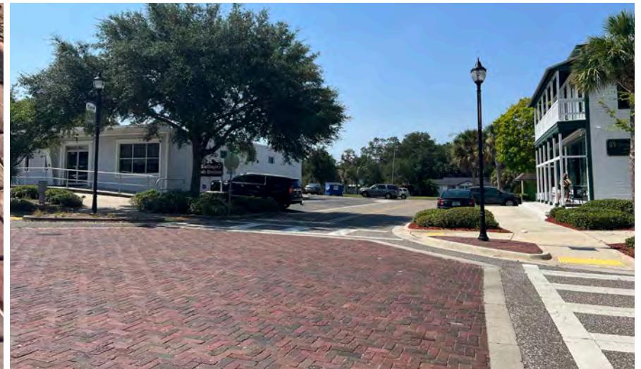
Existing Brick Intersections
