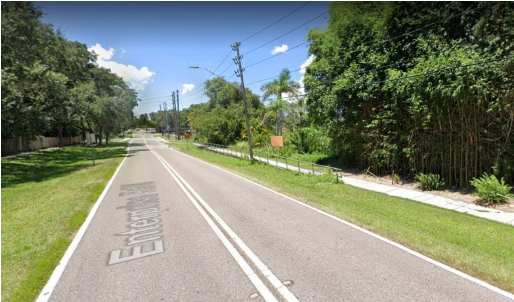
Looking northwest from Enterprise Road
