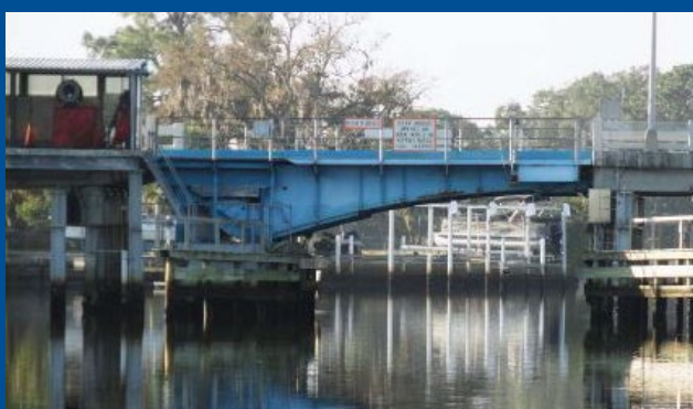
Above: Existing Narrow Sidewalk on Bridge
