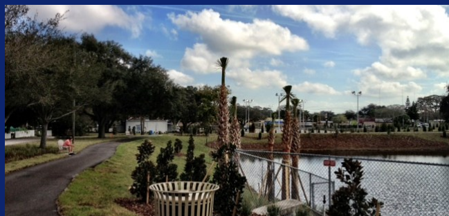
New Landscaping & Hardscaping improvements for stormwater ponds
