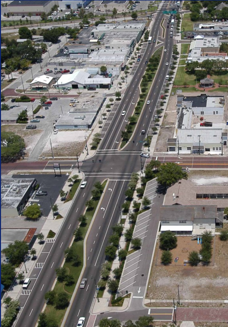
West Bay expansion and landscaping 2001
