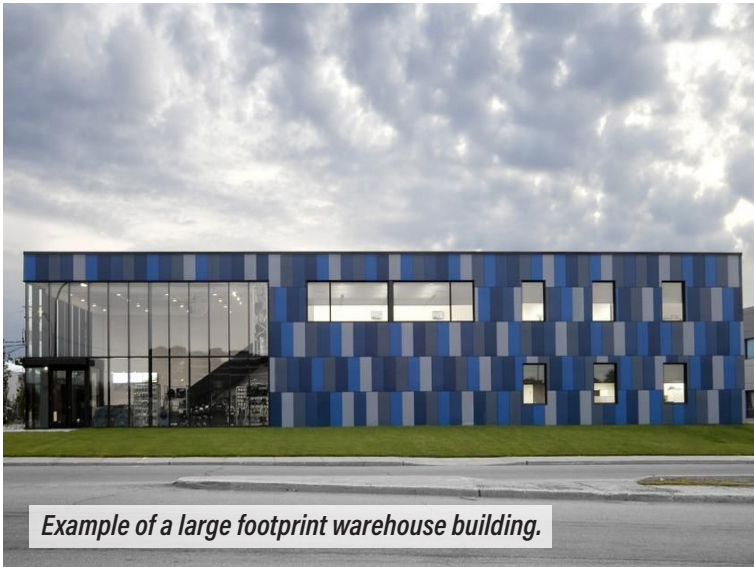
Large footprint building in a downtown setting.
