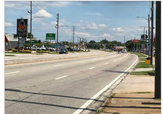
US 19 north of 62nd Avenue North
