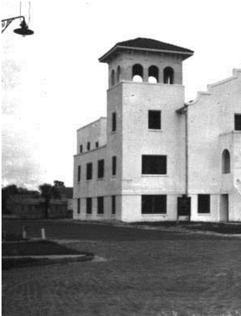
Photo 2a. Bell Tower Roof Before
