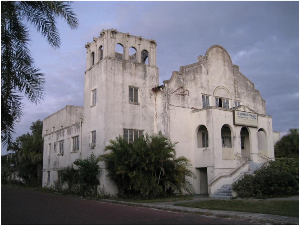
Photo 3a. Bell Tower Before
