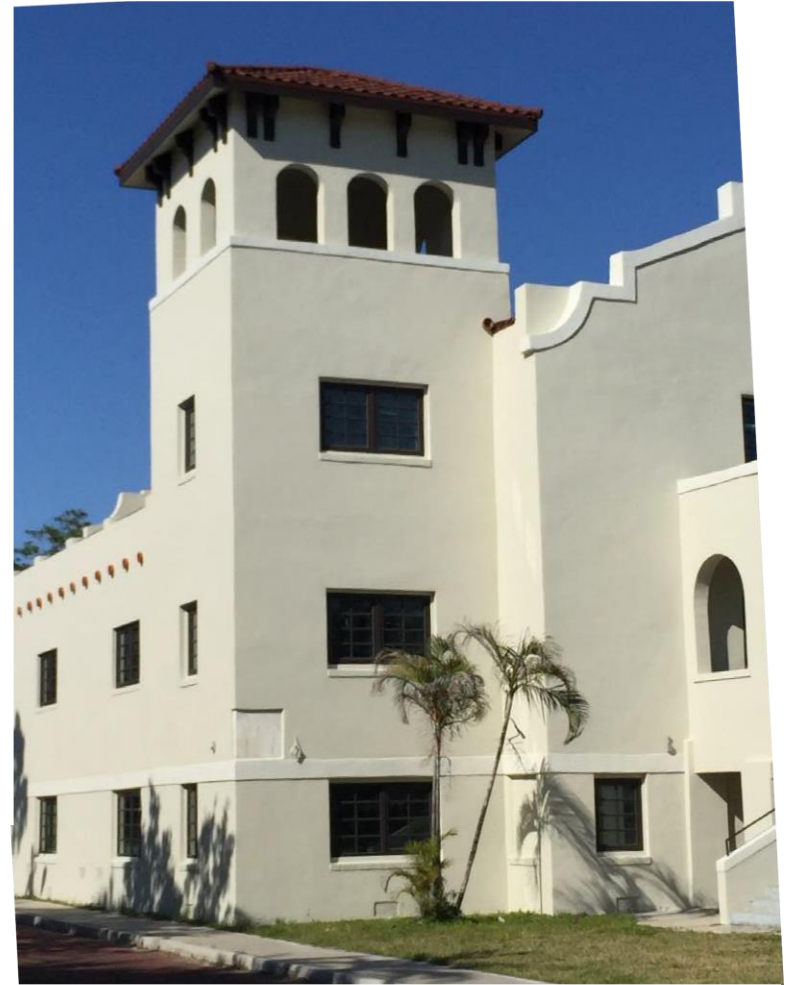
Photo 2b. Bell Tower Roof After
