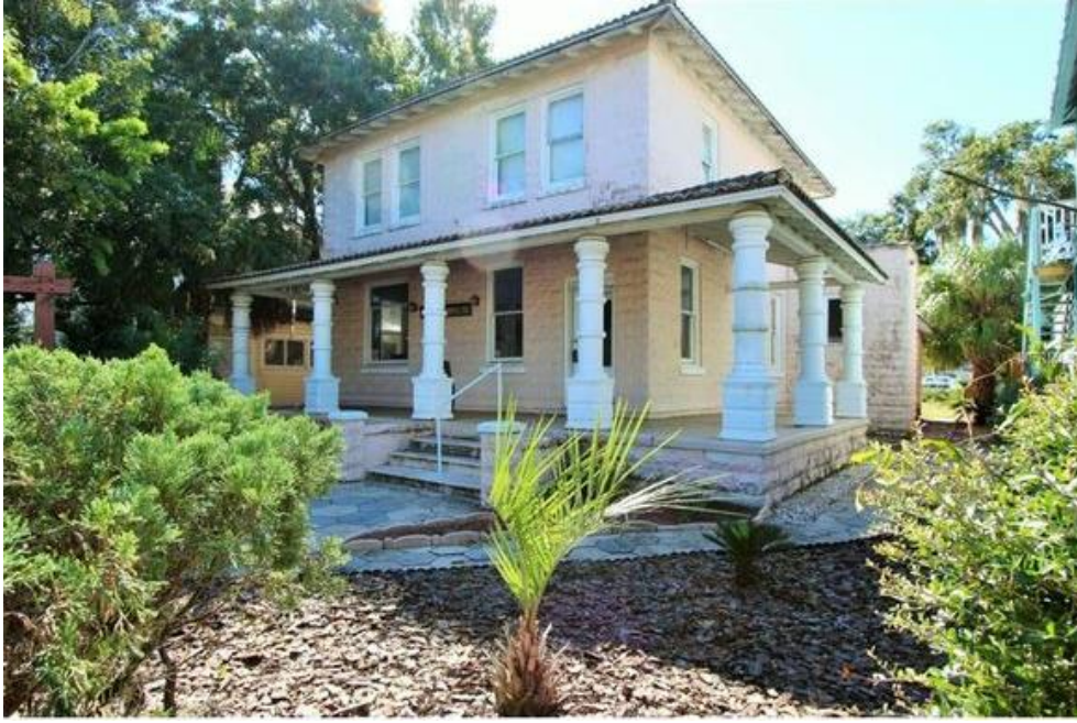
Photo 1a. Roof & Porch Before
