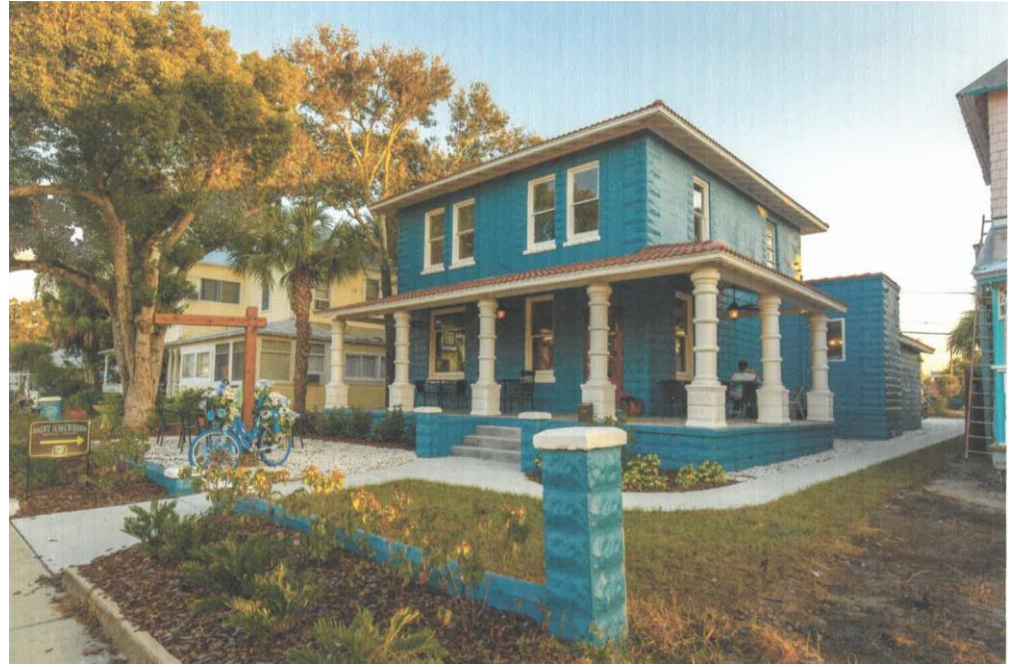
Photo 1b. Roof & Porch After
