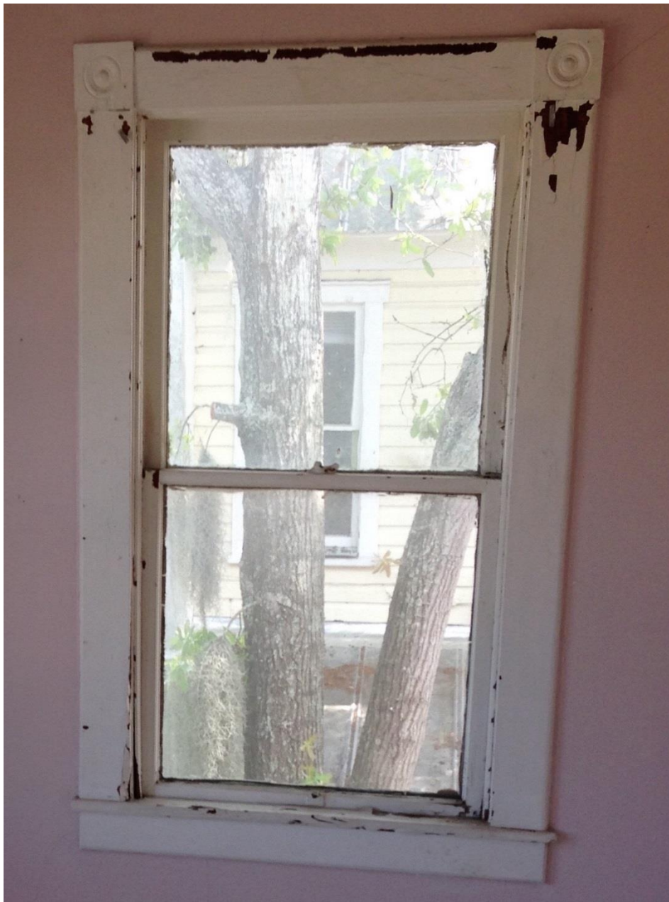
Photo 2a. Windows Before
