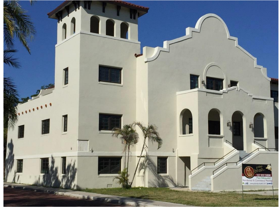
Photo 3b. Bell Tower After
