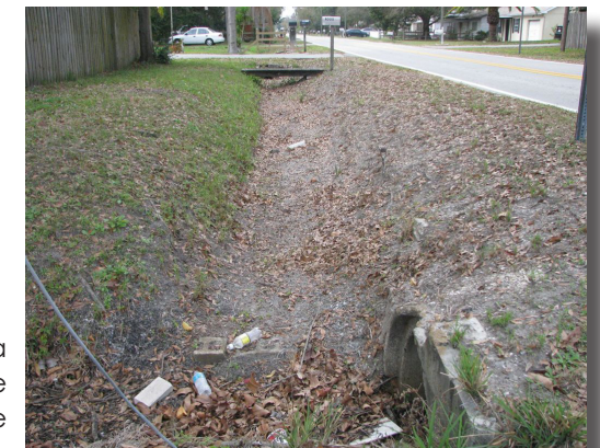
Existing Area Drainage Infrastructure
