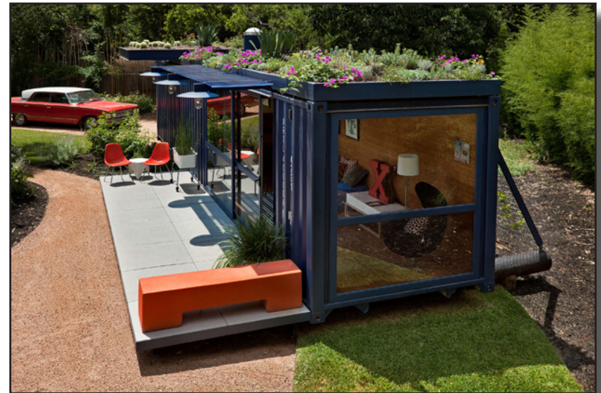
Container Guest House, Poteet architects, Ip, San Antonio, TX
