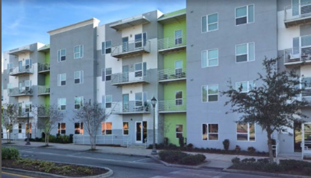
The Nolen, Clearwater, 39 units per acre
