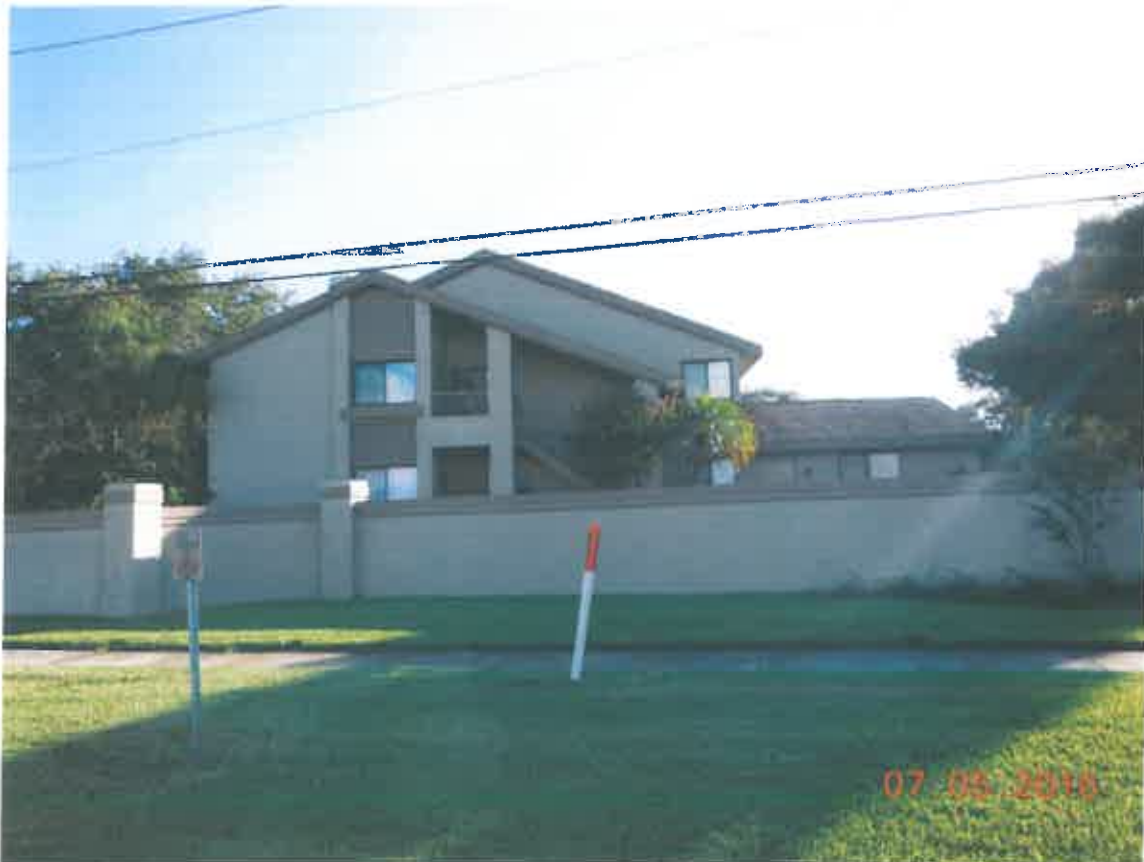
Photo 2B: Standing on West side of McMullen Booth, looking West towards Condo
