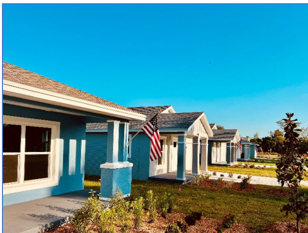
Habitat for Humanity for Pinellas and West Pasco Greenway Habitat homes in the Lealman CRA.
