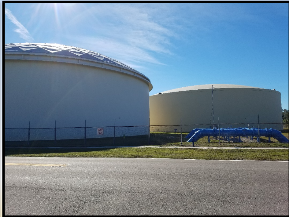
View of utility facility to the south
