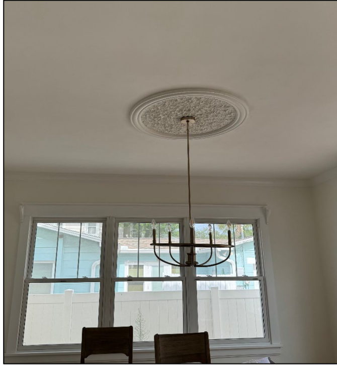
Figure 15: Restored plaster in dining room, post construction.
