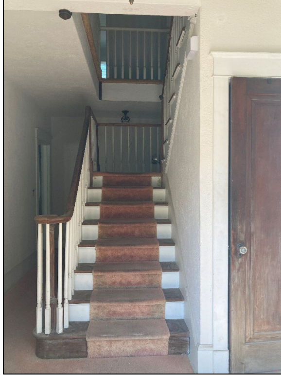
Figure 3: Front staircase, prior to construction
