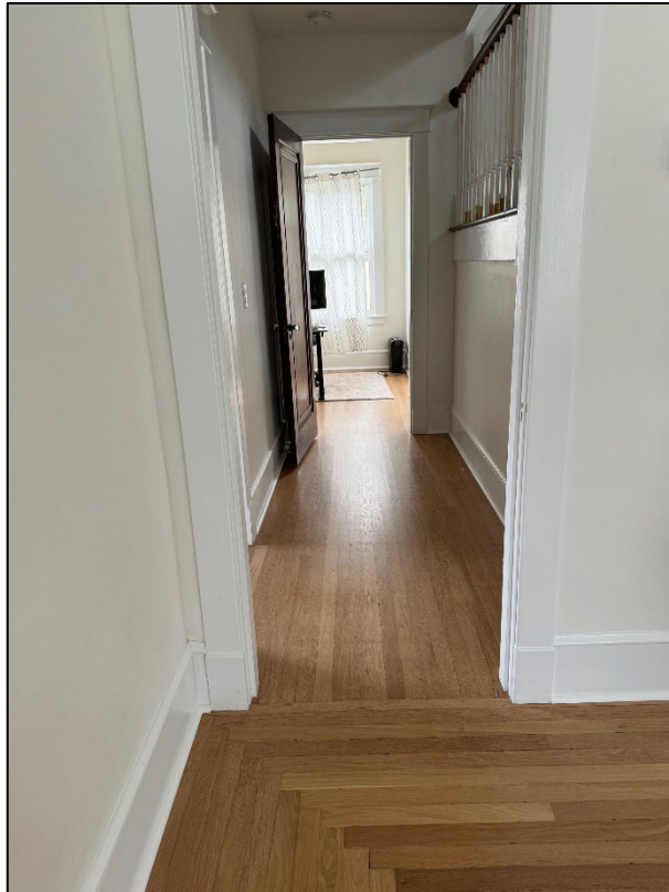
Figure 16: Restored wood flooring, post construction
