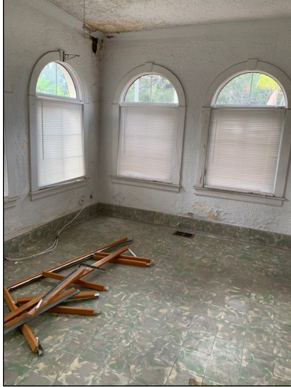
Figure 7: Family room, prior to construction
