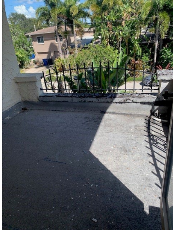
Figure 10: Roofing, prior to construction
