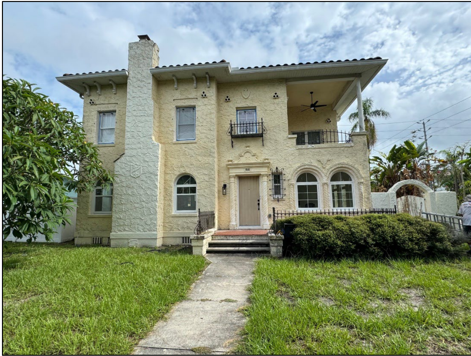
Figure 2: Front façade after rehabilitation.
