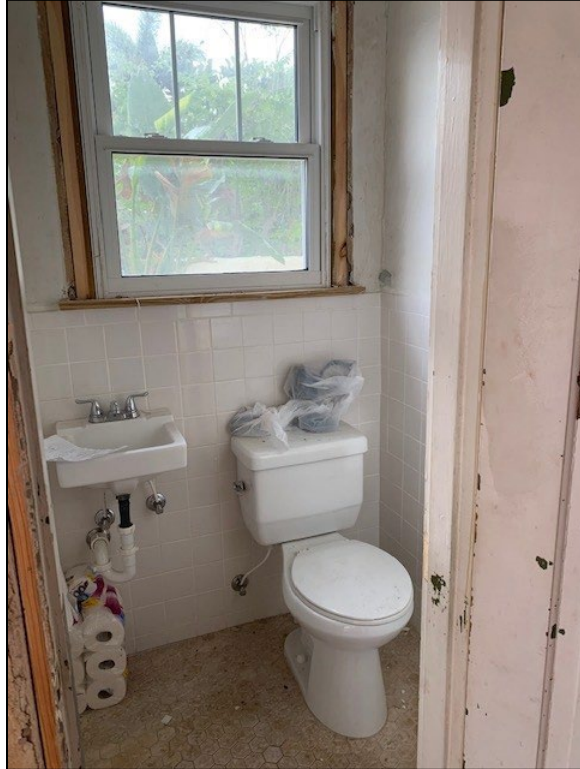
Figure 8: Bathroom, prior to construction
