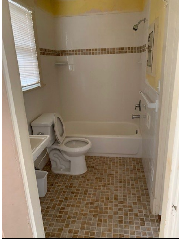
Figure 9: Bathroom, prior to construction
