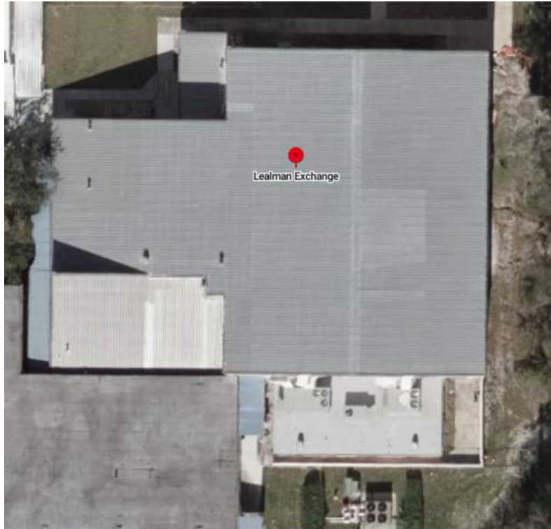
Photograph 1 – Overall Aerial Photo (Google 2023)
