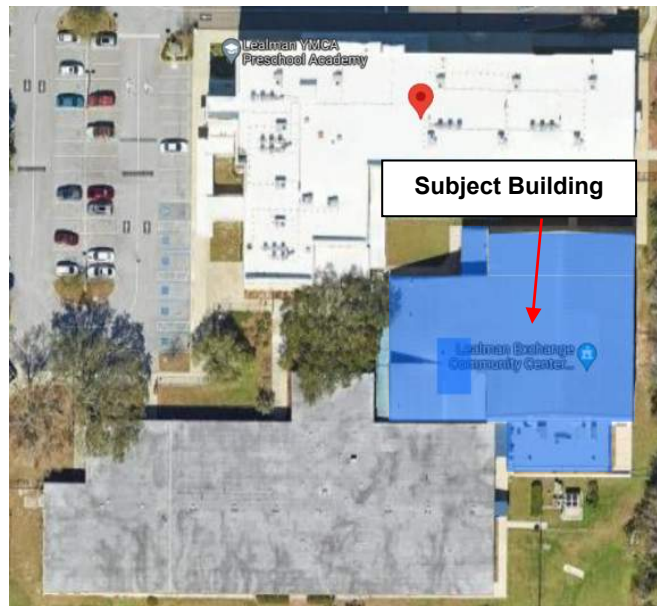
Figure 1-1 – Aerial Photograph Subject Building
