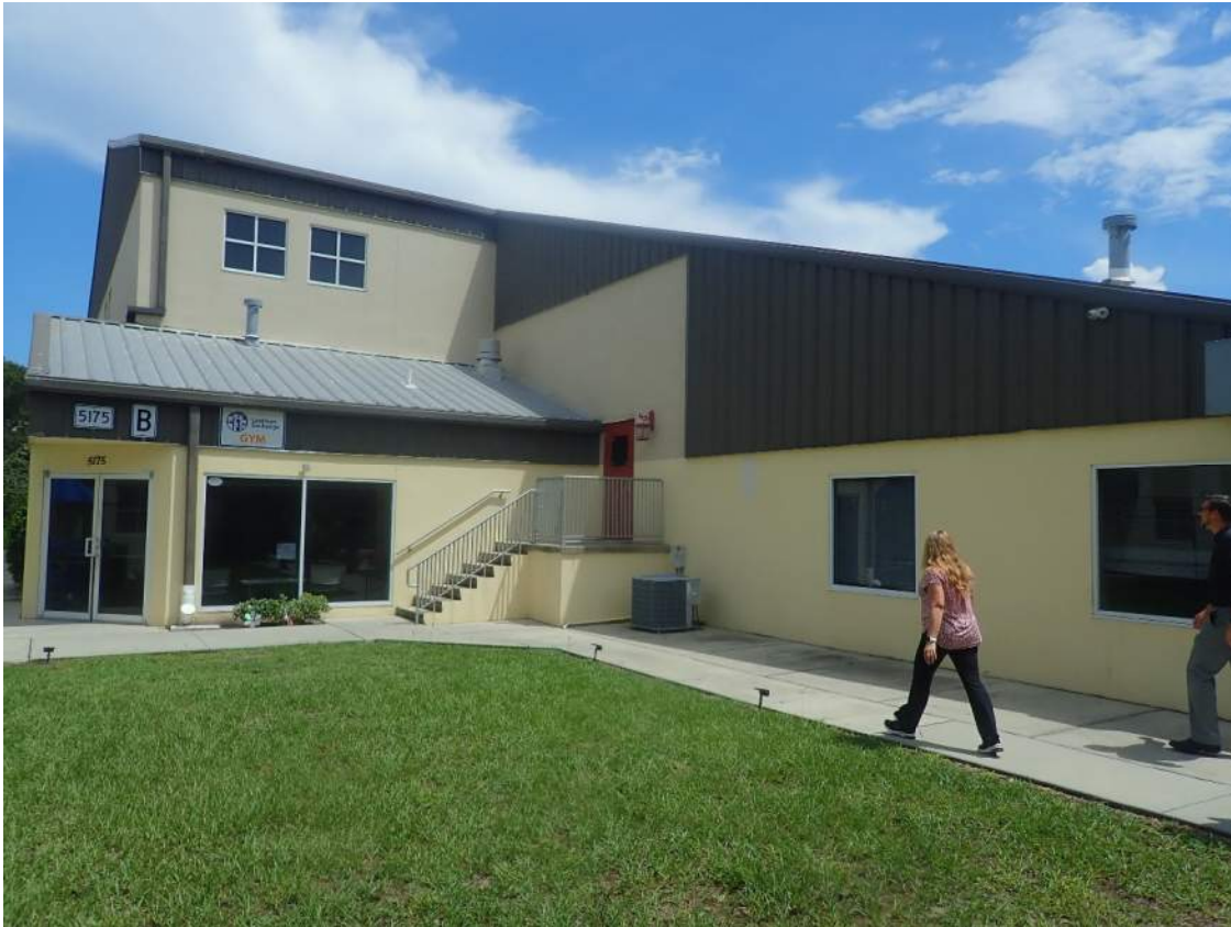
Photograph 3 – North West Elevation
