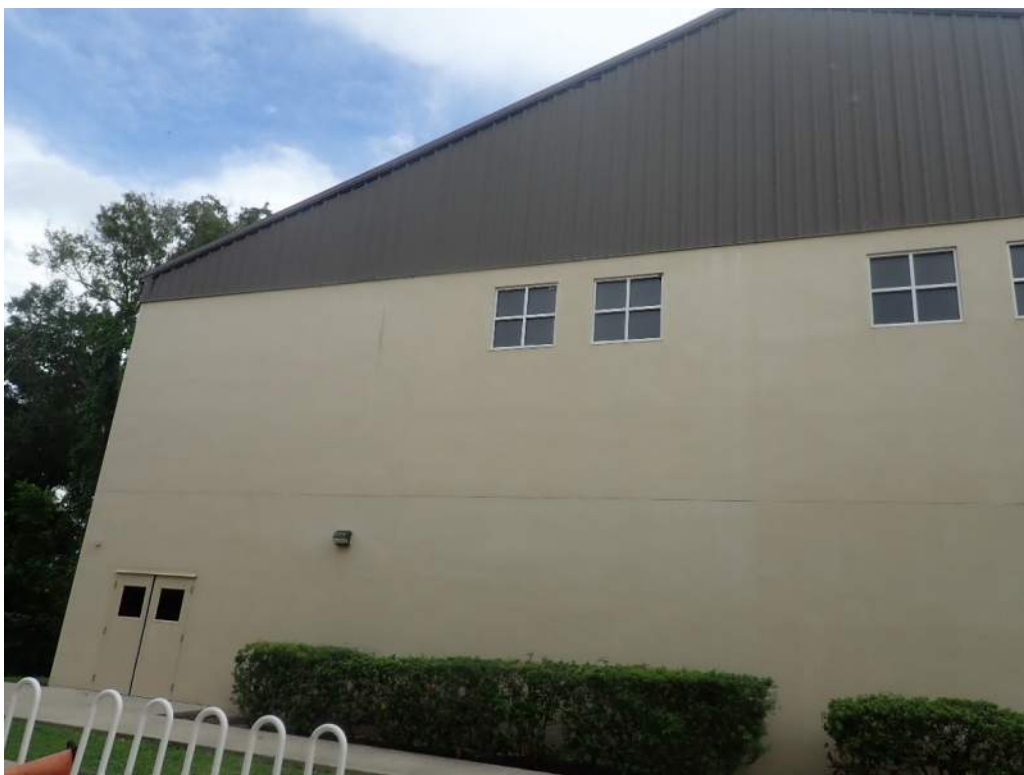
Photograph 4 – Partial North Elevation (Left side)
